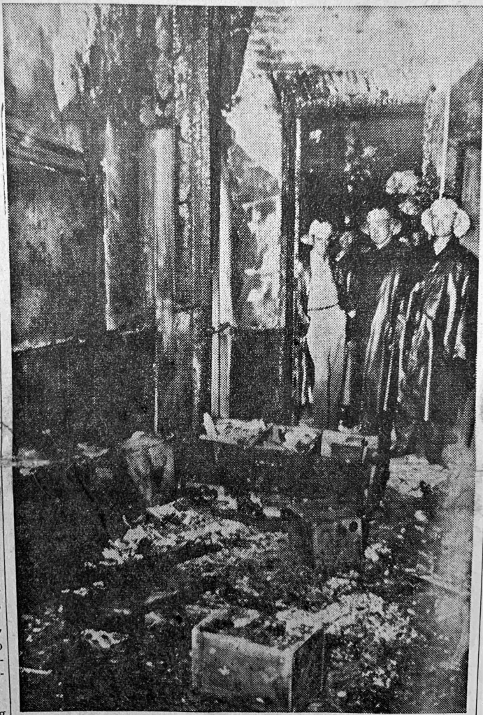
SEARED CLASSROOM —A portion of the interior of a classroom at the Lincoln elementary school is pictured shortly after the fire which struck the building early Monday. Two empty fuel cans were found inside this room. They can be seen in the foreground. The lock on the door at which the firemen are standing had been pried loose. Bookcases can be seen at the left and part of the pupil desks at the right. Firemen pictured, left to right, include Dave Higham, Ledger McConnaughey, Orva Harshbarger and Roger Faris, Sr. (Staff Photo)
