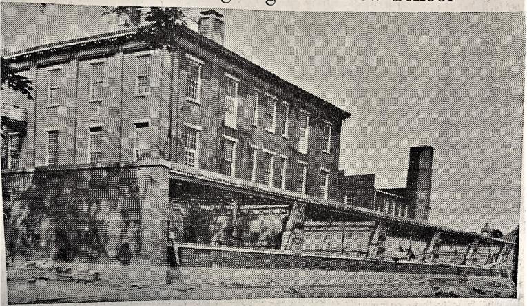
COMING IN ON WING—Interior walls are being completed on the south wing of the new Webster elementary school here. Roof joists are in place and windows have arrived and are ready for installation. The south wall of the wing, containing classrooms only, will have large window areas, overtion. The project is scheduled for completion in time for the fall term of school. (Staff Photo)
