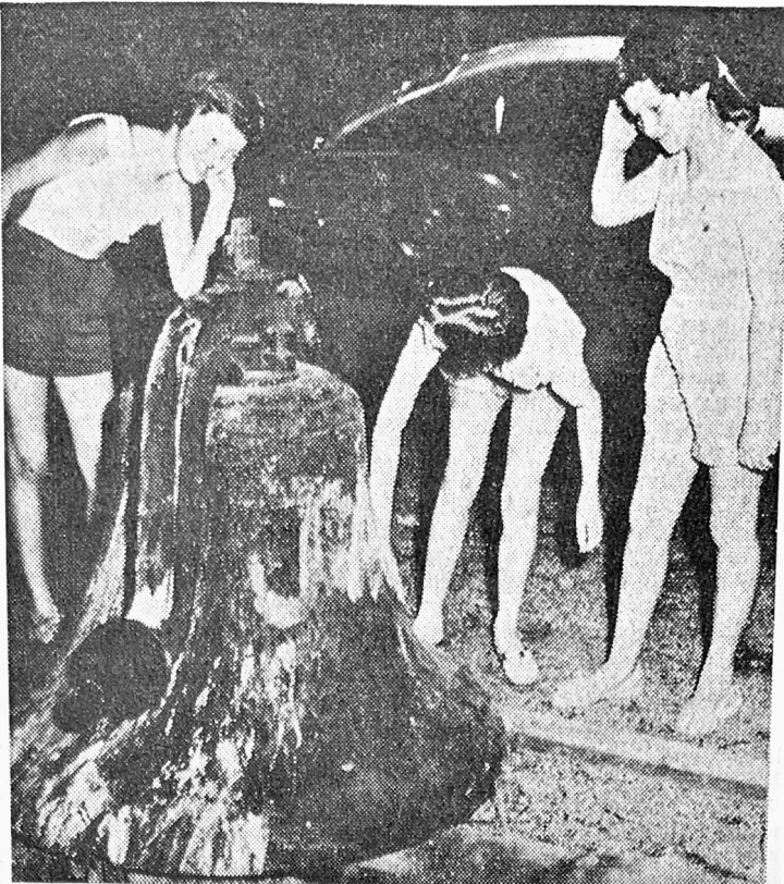
LAST RING —Paula Owens, center, taps the old bell from atop the Washington School, while her two classmates, Moisselle Shoemaker, left, and Diana Lemon give a listen. The bell was removed from the building last week by a demolition crew, preparing the Washington School for rebuilding. All three girls were in the fifth grade this past year and will have to hike across town to the Webster School this fall. The bell itself is a 44-inch steel-alloy church bell, made by the C. S. Bell Company here. It had hung in the Washington School since late 1896 or early 1897.
